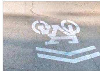
Shared lane markings also provide directional support for bicyclists.
