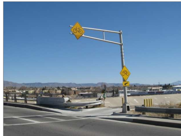
Type 1 crossings include signage and pavement markings.
