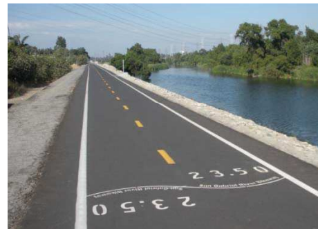
Pavement markings along the San Gabriel River Bikeway indicate mileage at quarter mile intervals.
